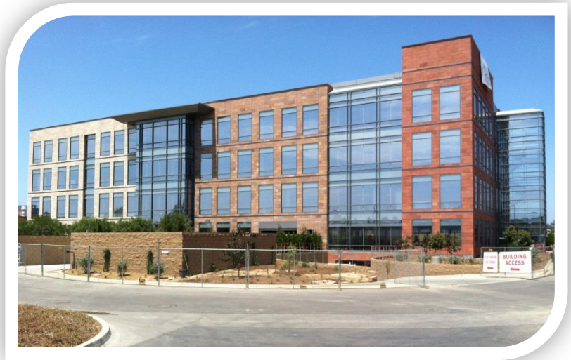
Figure 1: Exterior View of Research Facility Core and Shell
